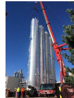
Installation of the CO 2 storage
